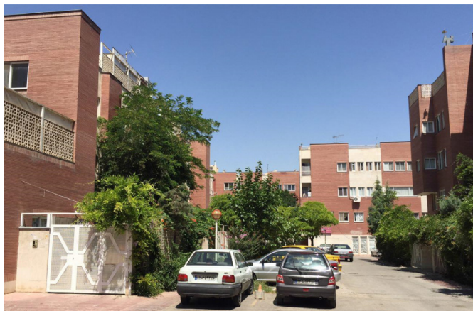
Figure 1 A general view of the surveyed area.
