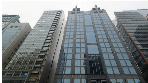
Figure 4 Gangnam Street: Building Facade
