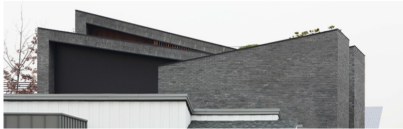
Figure 11 The Roof Scene (c)Wang, Kyutae , The Urban Landscape Made of Collective Masses (c)Kim, Jaekyung
