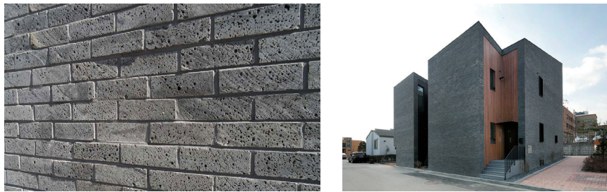
Figure 7 The Surface of Basalt Brick Wall, the Entrance Scene, Photo (c)Wang, Kyutae
