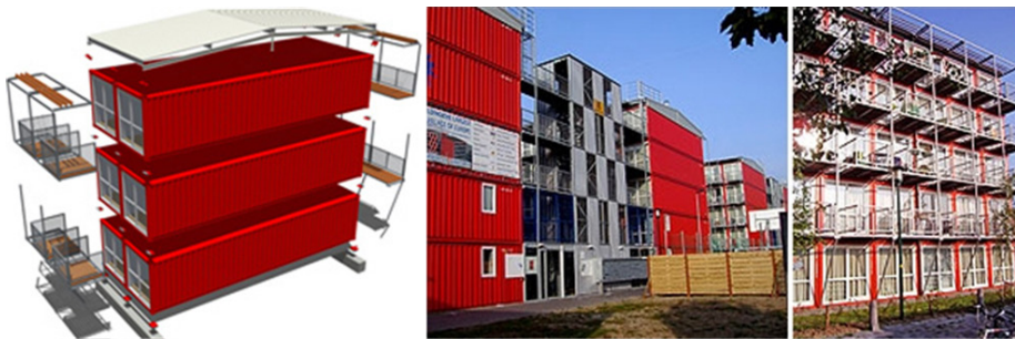
Figure 1 Module structure a dormitory keetwonen in Amsterdam
