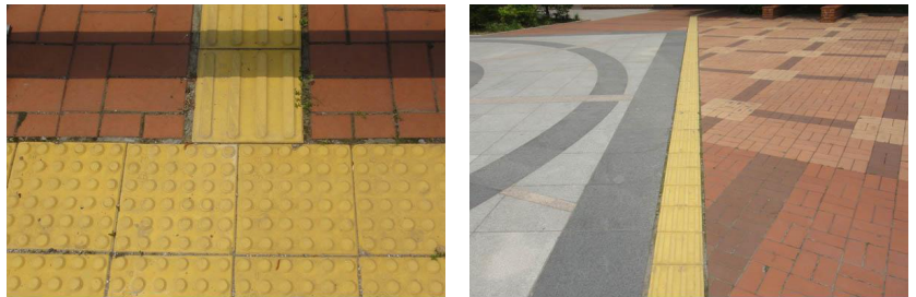
Figure 3 Road with braille blocks (warning block on the left, leading block on the right)
